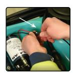
2) Mount the hose holders on either the front or the back of your sprayer using a phillips screwdriver.
